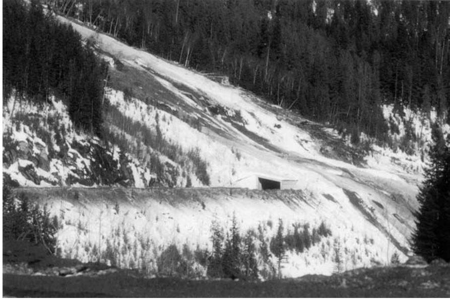
Figure 5. A snow shed protecting the Trans-Canada Highway at Rogers Pass, British Columbia. Photographer: C. Stethem.
