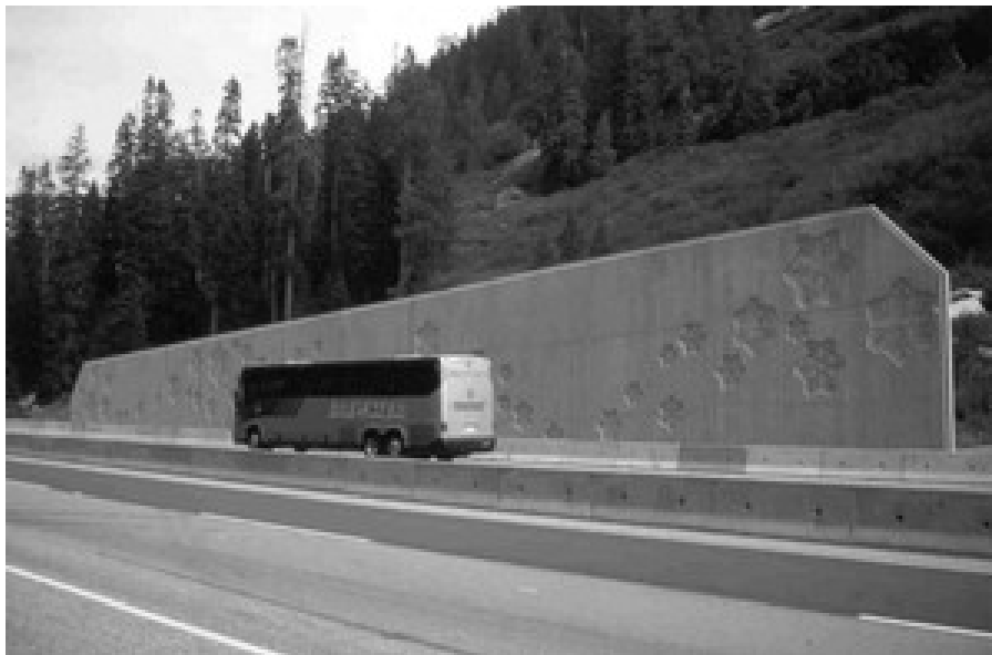
Figure 6. A reinforced concrete wall protecting Highway 5 near Coquihalla Pass in British Columbia. Photographer: British Columbia Ministry of Transportation Snow Avalanche Program.
