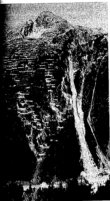
Figure 9.53. Progressive reforestation in avalanche terrain. Left, taken in 1907, shows masonry terraces for protection of planted forest; middle photo taken in 1938; right photo in 1957. (Photos from Swiss Federal Institute for Snow and Avalanche Research with the permission of Rhätische Bahn)
