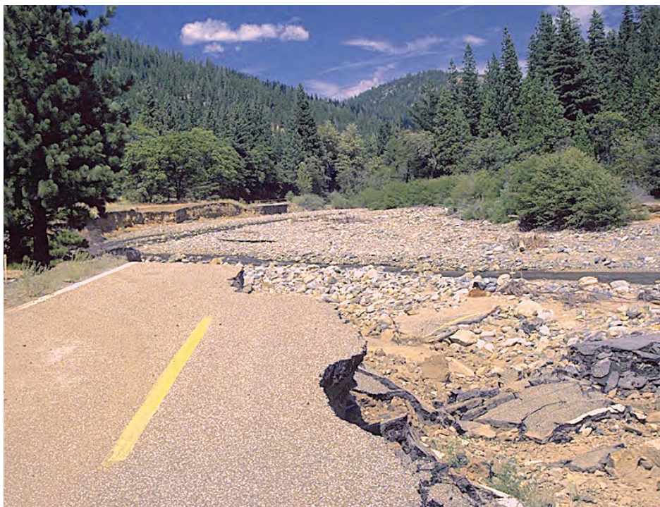
Figure 11.10 —Washout of a road in a floodplain as a result of channel widening during high river flow (photo from Keller and Ketcheson 2015, used with permission).
