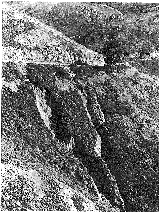
FIGURE 8.5.—If road drainage becomes concentrated, it must be discharged into places that can handle the flow without accelerated erosion. When the natural drainage of small streams is changed and concentrated flow is discharged into nondrainage areas, severe gullying and landslides can result.
