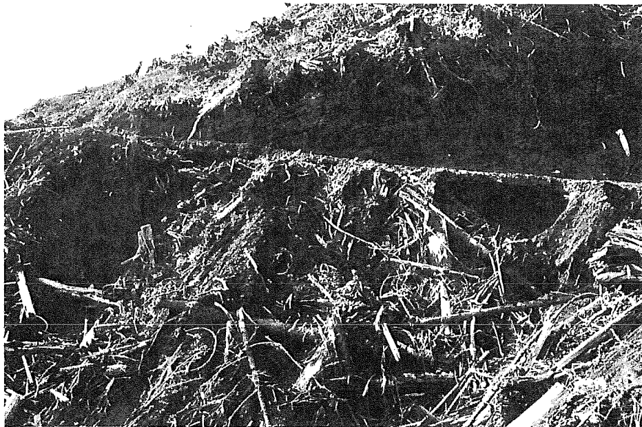
FIGURE 8.7.—Incorporation of woody debris into road fill and sidecast material inevitably leads to mass failure and surface erosion.
