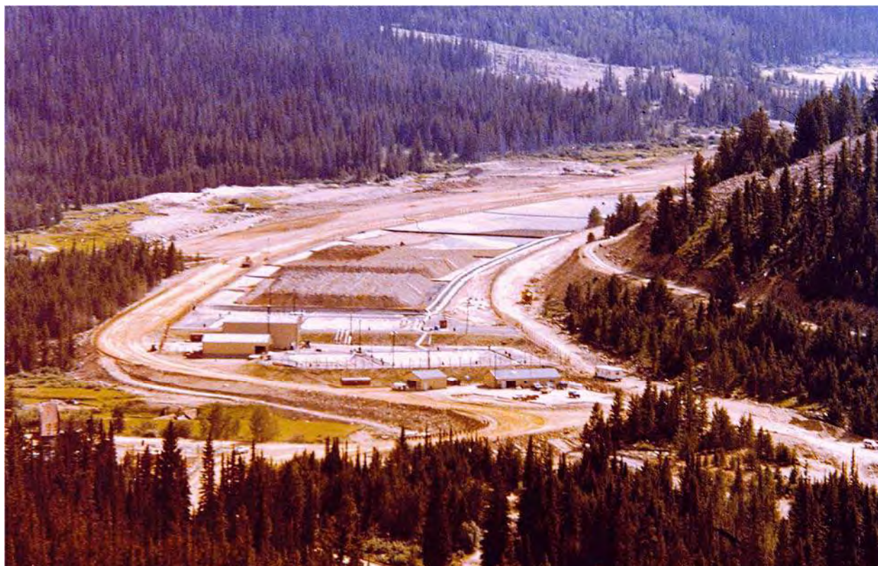
Figure 6.3: Canadian Superior Mining (U.S.) Ltd. Heap Leach Processing Facility
