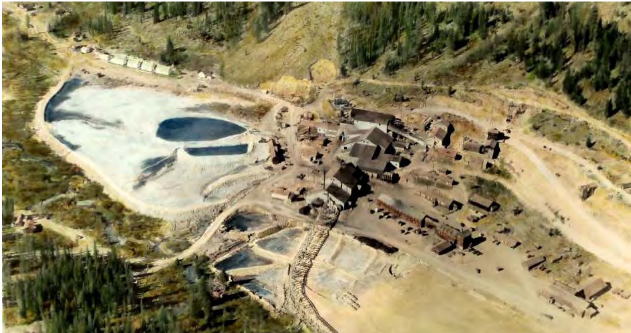
Figure 6.1: Bradley Mining Company Processing Plant and Tailings Pond
