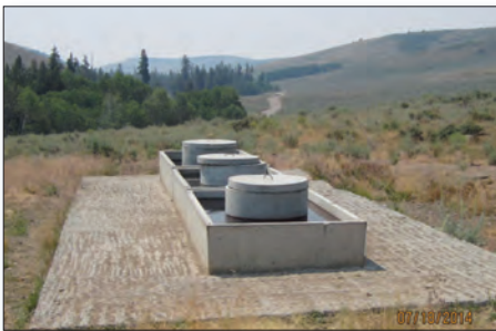
Figure 2. Project partners installed alternate water sources to keep livestock away from Shoshone Creek.
