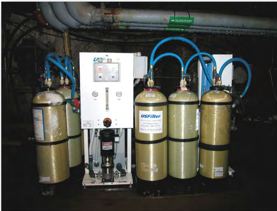
Figure 19: In-Mine Ion Exchange Treatment System at the Soudan Mine
