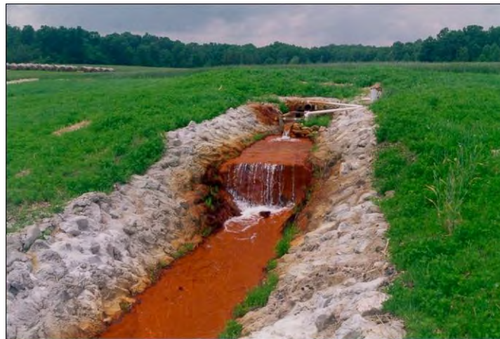
Figure 2: Anoxic Limestone Drain Outflow at the Midwestern Reclamation Site, Pike County, Indiana
