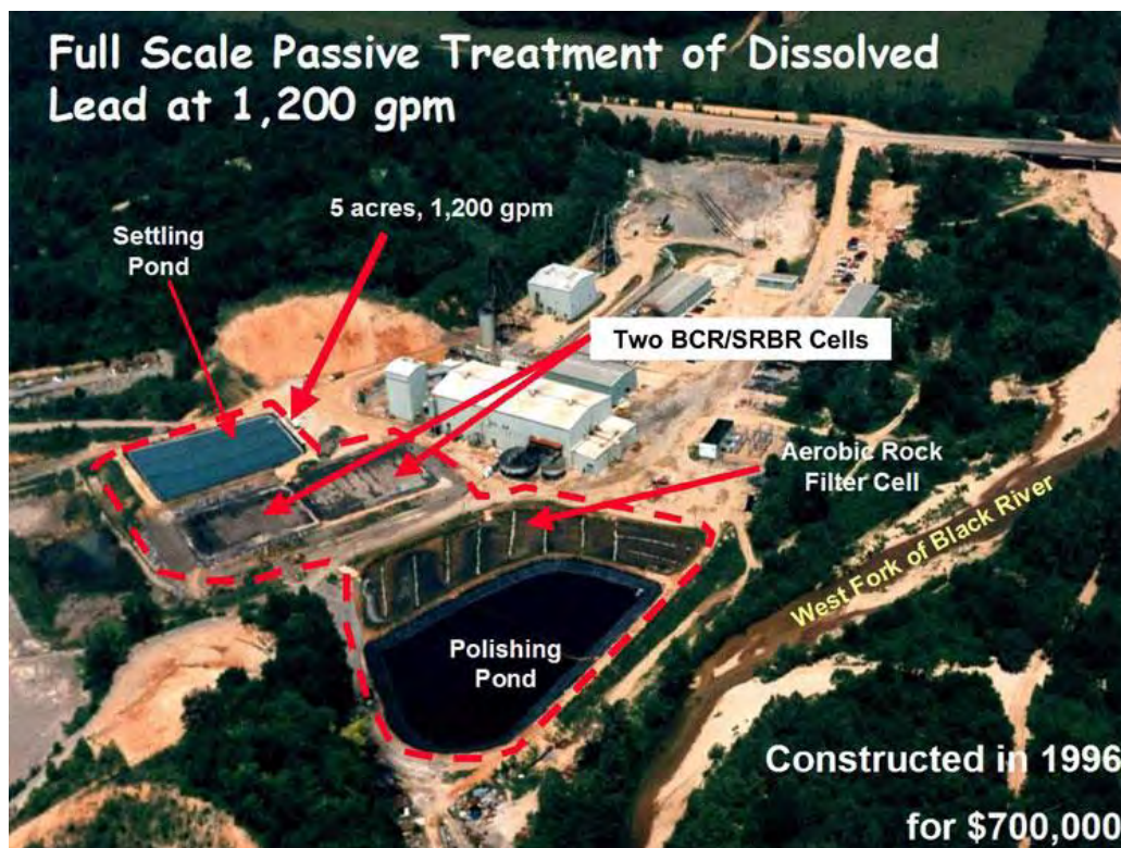
Figure 7. Example of Passive BCR System
