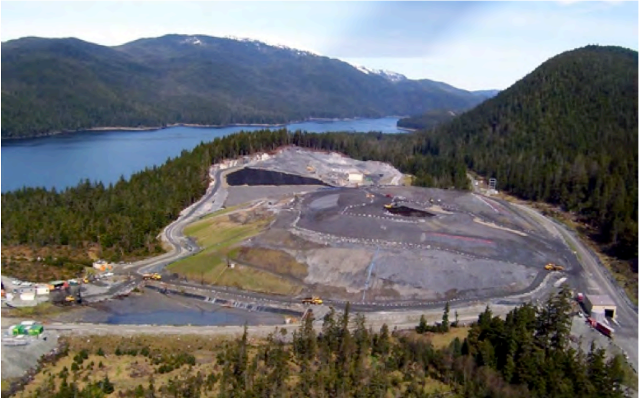
FIGURE 9.1.1 FILTERED TAILINGS FACILITY, GREENS CREEK, ALASKA
