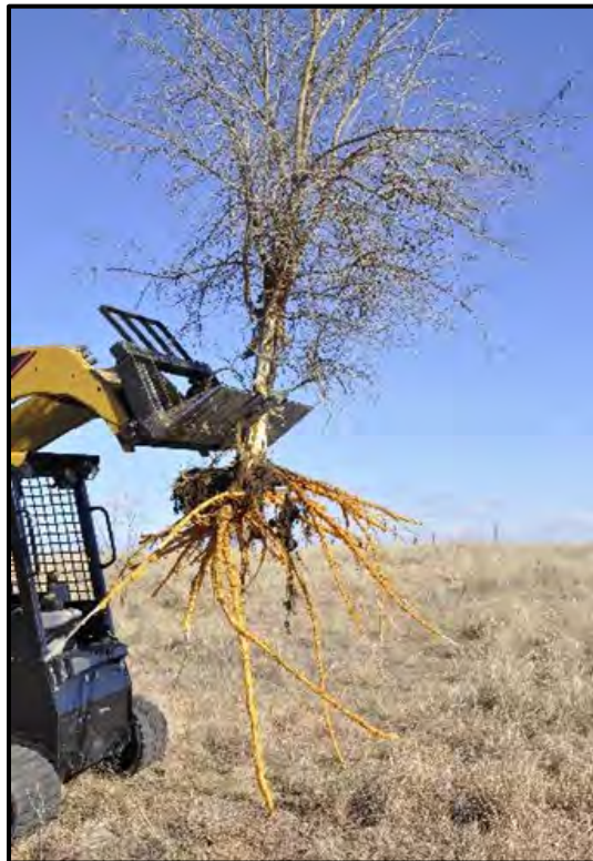
Figure 2-12. Example of tree plucking.
