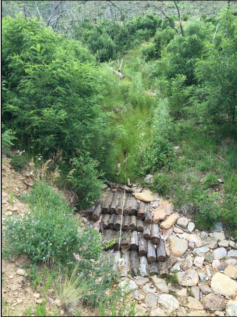
Figure 2-17. After: The restored large headcut on the Cibola National Forest, 2 years after restoration was implemented with a log drop.
