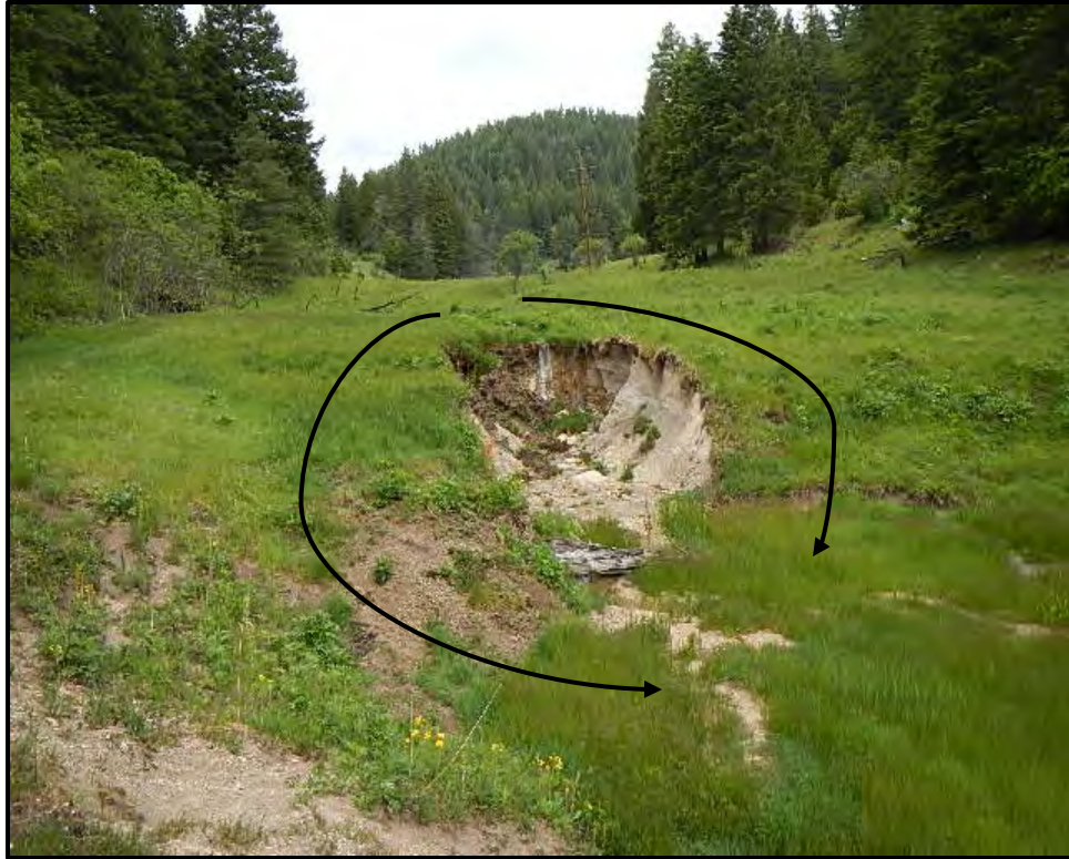
Figure 2-18. Illustration of where ditches may be constructed on either side of the channel, redirecting flow around the headcut to flow back into the channel below the headcut.
