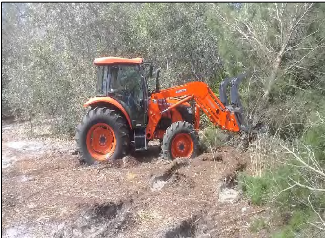
Figure 2-3. Example of tree pushing.
