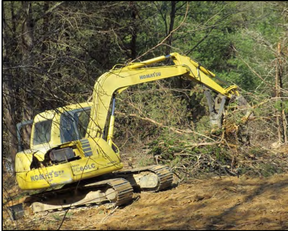
Figure 2-10. Excavator piling slash.
