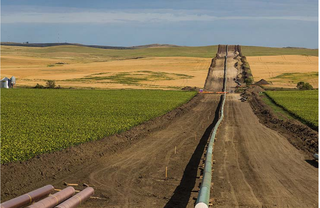
Construction on the Dakota Access pipeline near New Salem, N.D., in 2016. Tony Webster/Flickr
