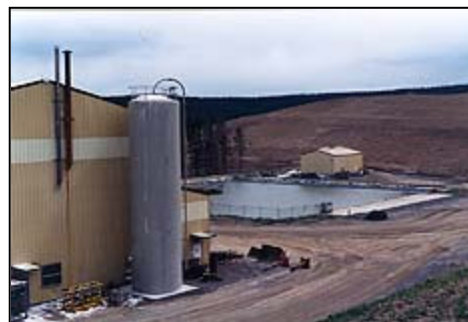
Water treatment facility at Beal Mountain Mine.
