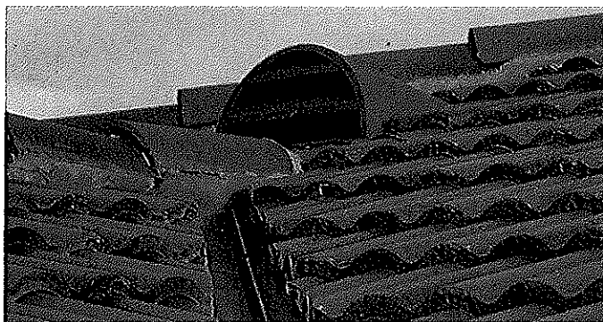
Reduce vent space to the bare minimum. Minimal gable-end vents (photo above) and dormer-type roof vents (photo below) are adequate to ventilate the roof of this Pacific Coast house. Soffit vents are eliminated altogether. The reduced venting meets code for the area because of the greater concerns for fire safety. Behind the vents, 1/2-in. wire mesh was installed to cut the risk that cinders would be drawn into the attic space.
