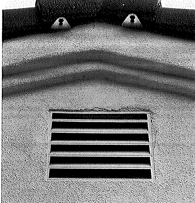
Reduce vent space to the bare minimum. Minimal gable-end vents (photo above) and dormer-type roof vents (photo below) are adequate to ventilate the roof of this Pacific Coast house. Soffit vents are eliminated altogether. The reduced venting meets code for the area because of the greater concerns for fire safety. Behind the vents, 1/2-in. wire mesh was installed to cut the risk that cinders would be drawn into the attic space.
