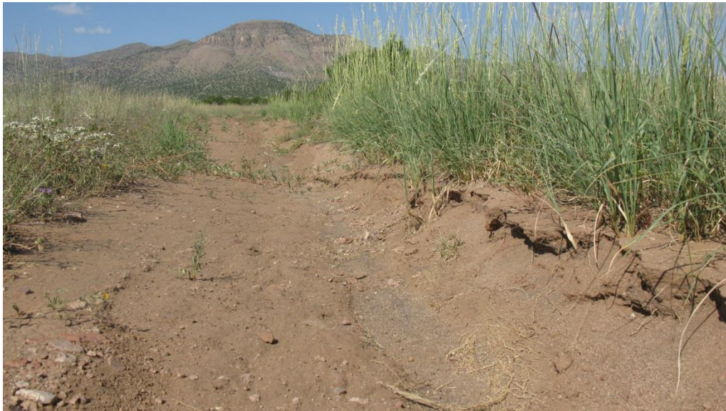
Figure 5. Heavy erosion after summer rains on track to the basecamp (same general view as Figure 1 above). This violates the Temporary Special Use Permit paragraph 22.
