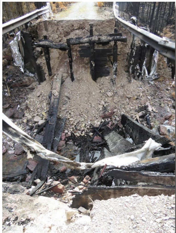
Wildfire burned this Road 549 bridge over Bunker Creek in 2015, stranding 3 bridges and 30 culverts beyond!
