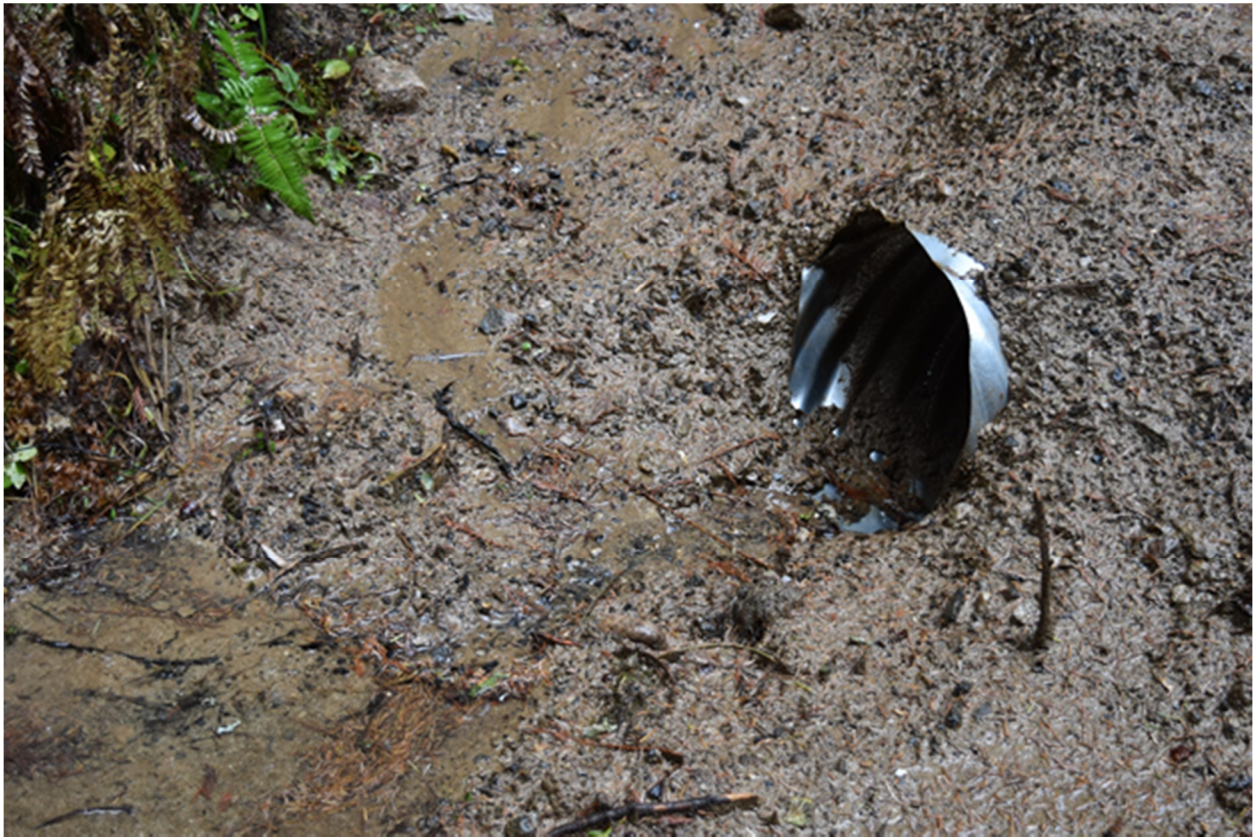
Below is a second culvert in that same area, conducting sediment:
