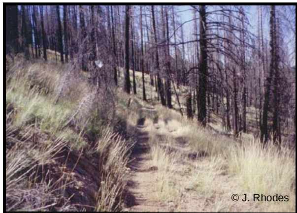
Photographs 2a & 2b. An example from Karr et al. (2004) of some of the typical impacts of the reconstruction of unused roads on vegetation, soils, road runoff, and sediment production. The left photo (2a) shows an unused road in 1996 on the Malheur National Forest, OR, which had undergone some recovery of vegetation and soil conditions through non-use, resulting in revegetation and reduced erosion and runoff. The right photo (2b) shows how reconstruction of the same road for MFT had reversed this recovery in 1999, increasing soil erosion and sediment delivery by surface runoff to a tributary of a stream inhabited by steelhead trout (listed as threatened under the Endangered Species Act at the time of photo). Such increases in sediment delivery lower the survival rates of steelhead and other aquatic species and degrade water quality, as discussed in the text. Photographs: J. Rhodes.
