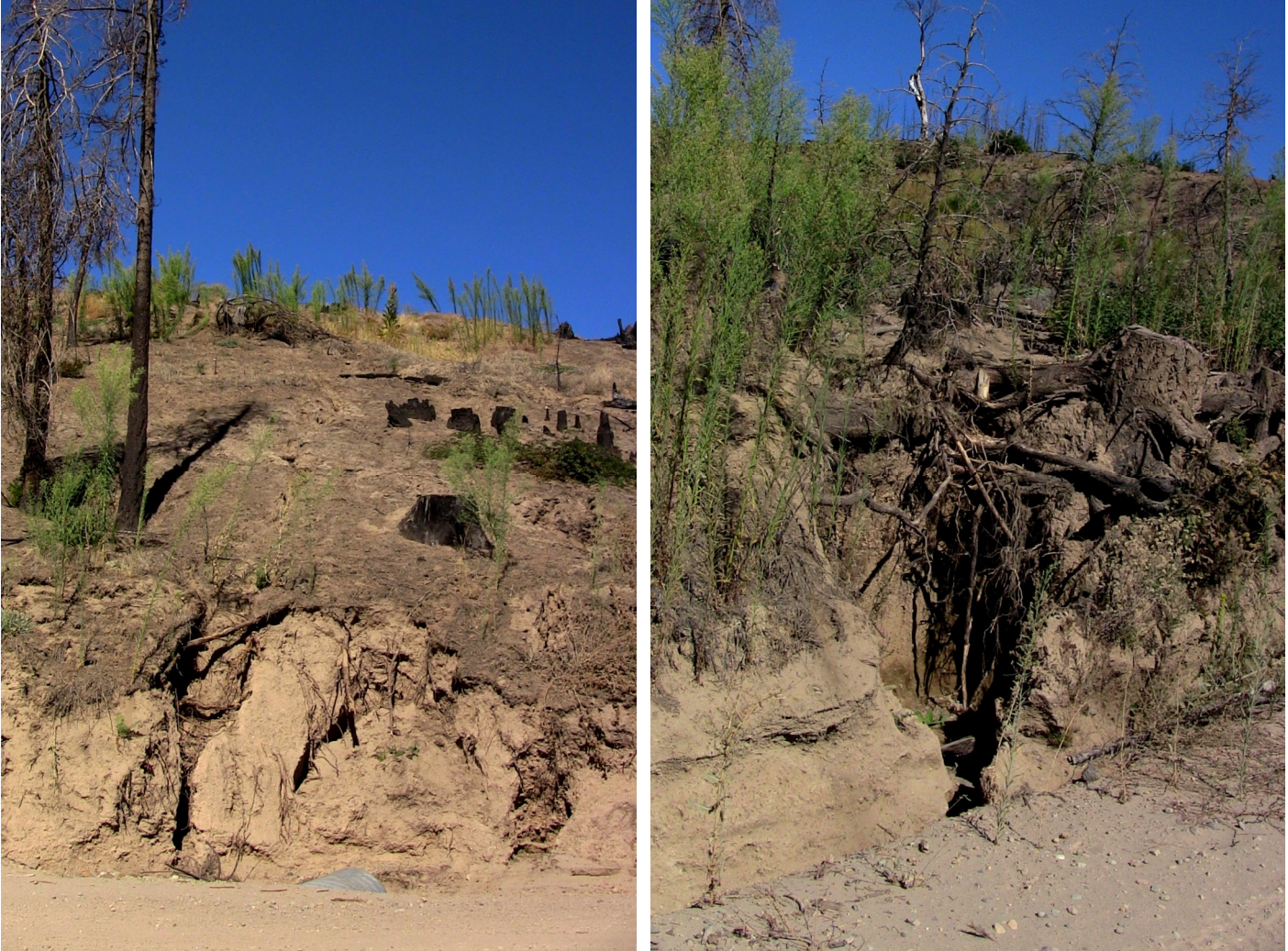
Figure 16. Roadcut bank erosion initiated or aggravated by overland flow from harvested areas upslope, September 2014.
