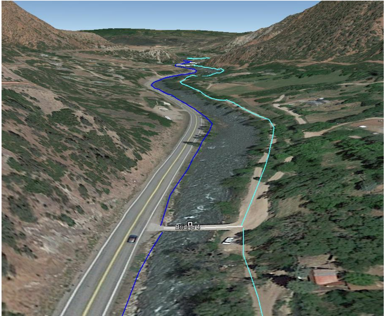
Figure 8 Existing bridge on a confined reach between the Red Wind Point and Nettle Creek sections. Alignment B uses follows the abandoned rail line, portions of which have been repurposed as roads, through the Nettle Creek segment.
