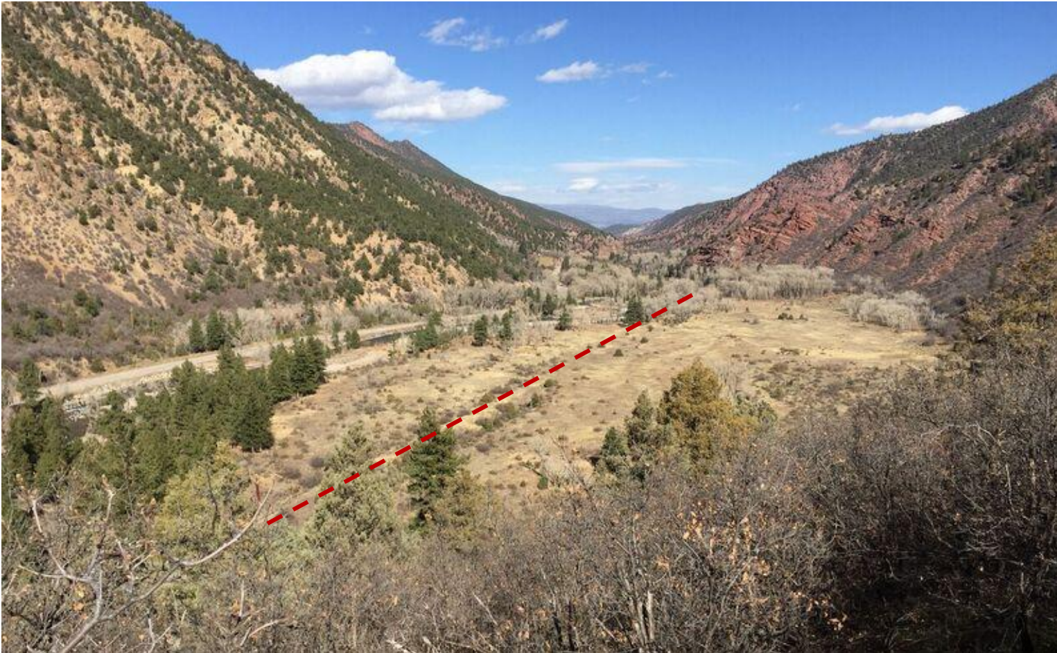
Figure 20 For Alignment B on the Janeway North section, a 10-foot-wide paved path would be constructed on the abandoned rail line that runs through the middle of the wide riparian area east of the river.
