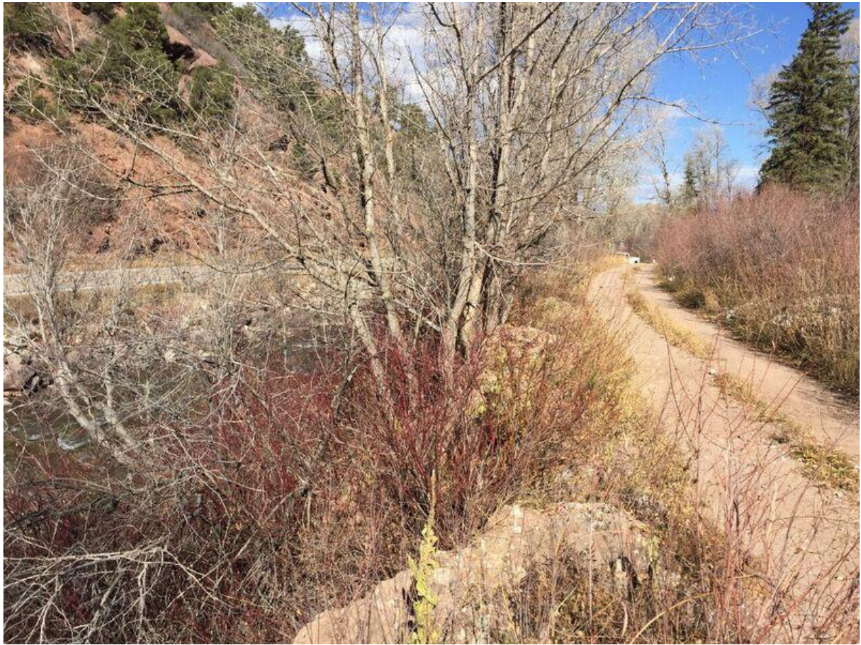
Figure 22 The rail line east of the river on the Red Wind Point section is now used as an un-surfaced access road that isolates the floodplain and riparian area (right) from the river (left). For Alignment B, a paved path would be constructed.
