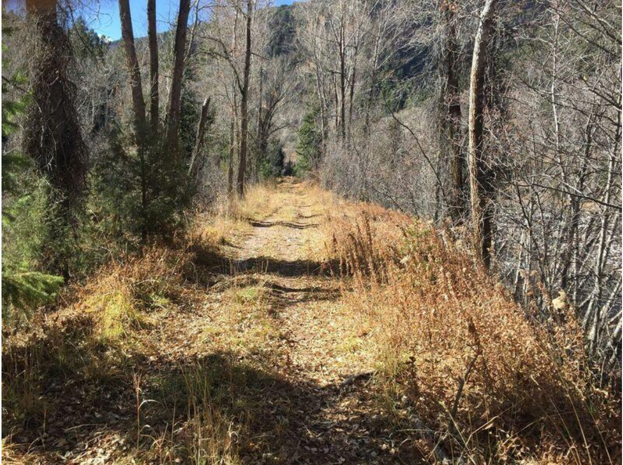
Figure 23 Another section of the rail line upon which a paved path would be constructed for Alignment B on the Red Wind Point section. The rail line fill cuts off the floodplain and riparian area from the river. Constructing a paved path would introduce significant impacts and probably eliminate any future opportunity to restore connectivity.
