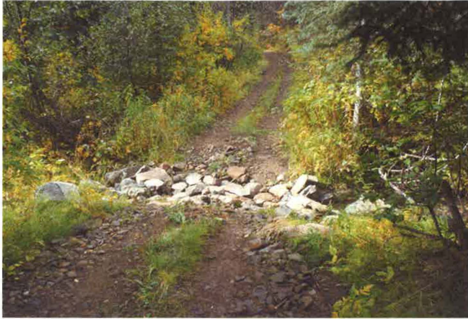
Figure 2. An example of stream crossing hardening that was performed as a restoration partnership project between the Forest and Tribe in 2014-15.
