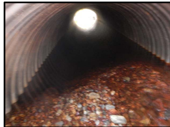
Culvert barrel, looking downstream 2017
