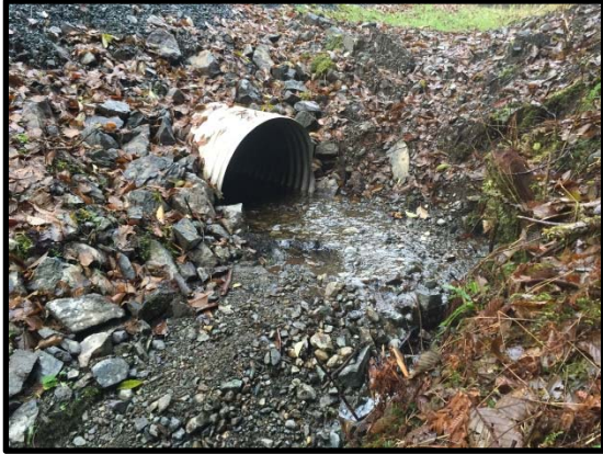
Culvert outlet, looking upstream 2015
