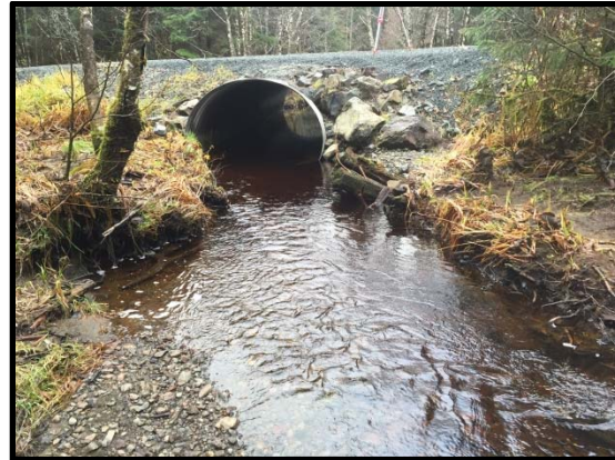
Culvert inlet, looking downstream 2015
