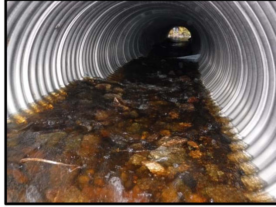
Culvert barrel, looking downstream 2015
