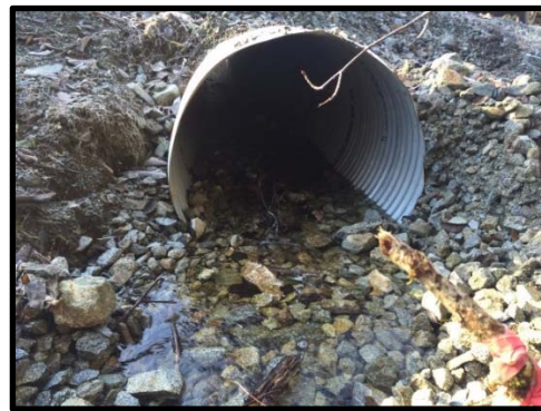
Culvert inlet, looking downstream, 2015
