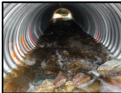
Culvert barrel, looking downstream 2015
