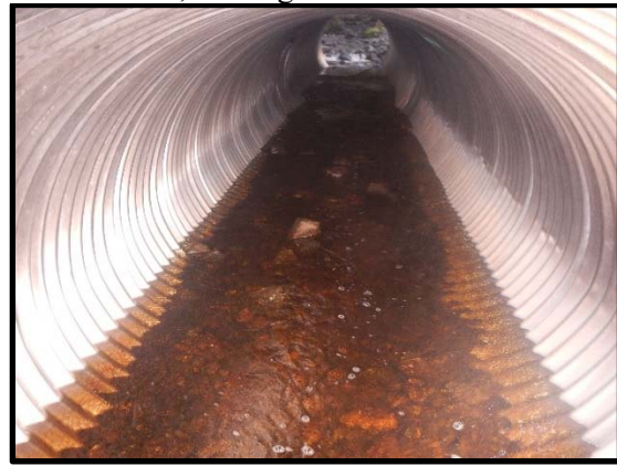
Culvert barrel, looking upstream 2017
