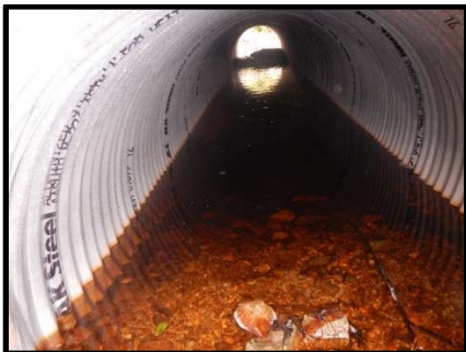
Culvert barrel, looking upstream 2017
