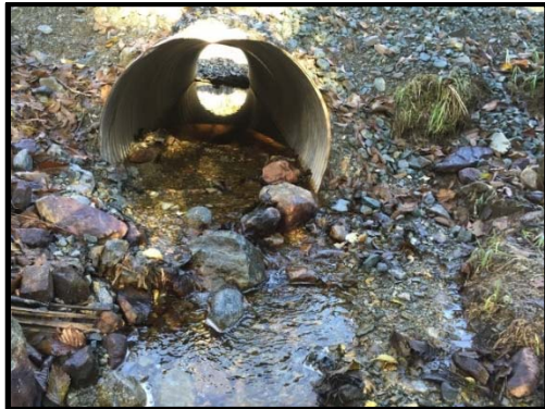
Culvert outlet, looking upstream, 2015
