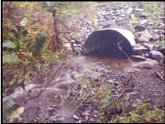
Culvert outlet, looking downstream, 2014
