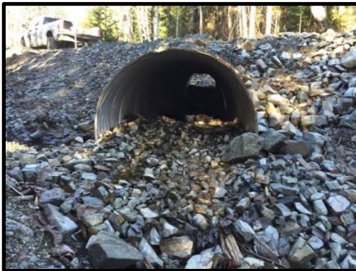
Culvert outlet, looking upstream 2015
