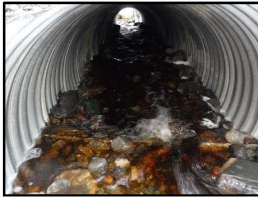
Culvert barrel, looking downstream 2015
