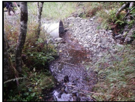
Culvert inlet, looking downstream 2017
