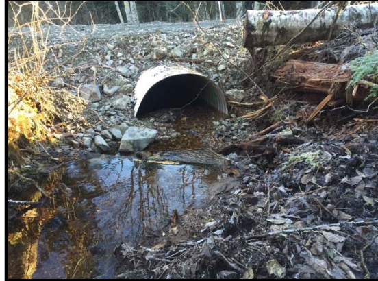
Culvert inlet, looking downstream 2015
