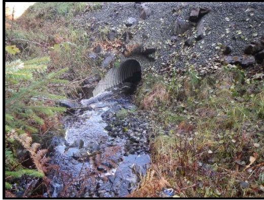
Culvert inlet, looking downstream 2017
