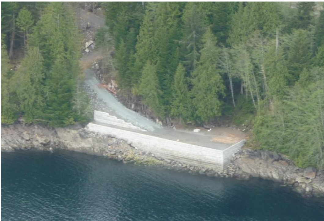
Access road and site pad- prior to completion, May 2010
