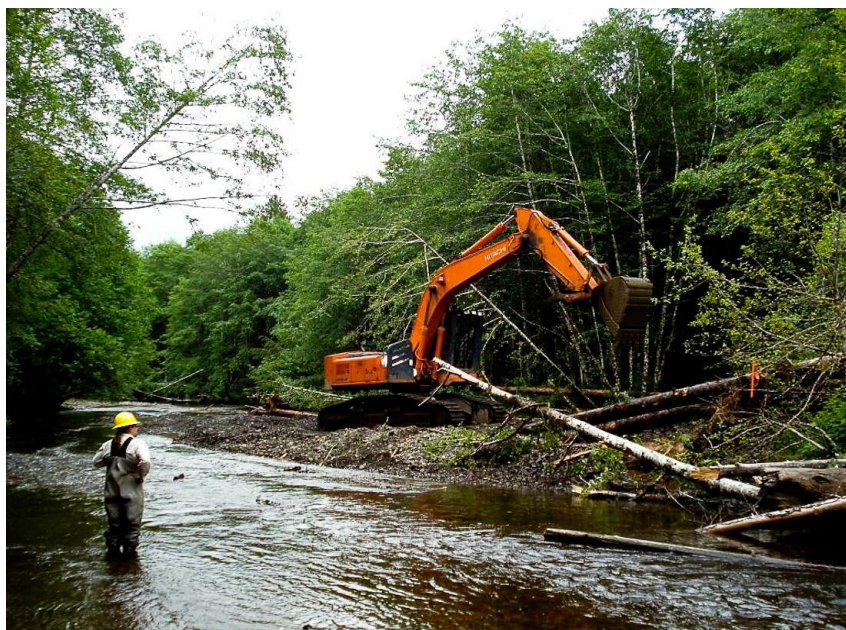
Watershed restoration project adds wood to stream to create fish habitat.
