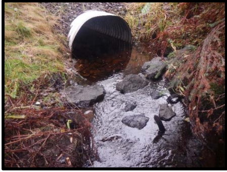
Culvert outlet, looking upstream
