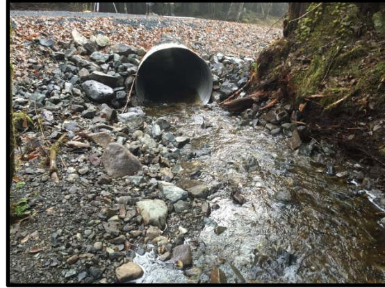
Culvert inlet, looking downstream 2015
