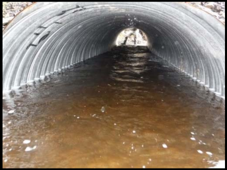
Culvert barrel looking upstream
