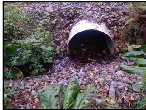
Culvert inlet, looking downstream, 2017
