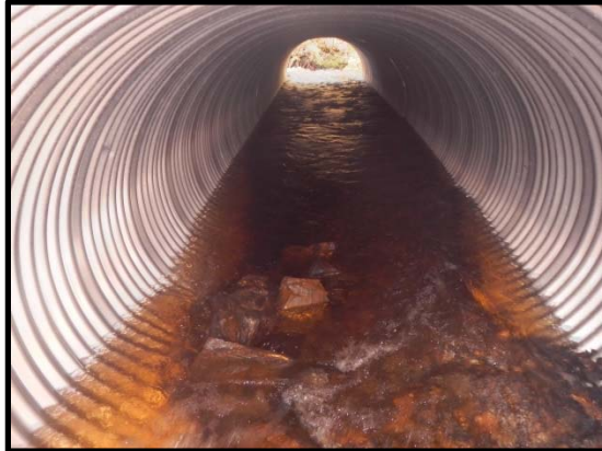
Culvert barrel, looking downstream
