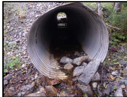
Culvert outlet, looking upstream 2017
