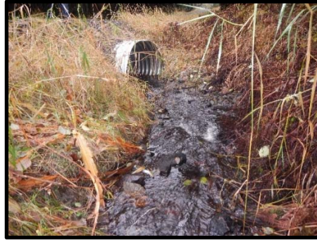
Culvert inlet, looking downstream 2017
