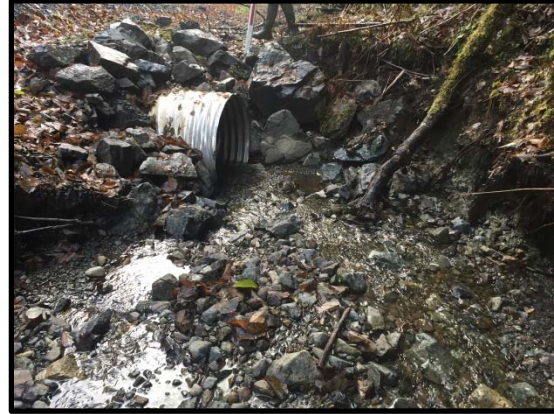
Culvert inlet, looking downstream 2015
