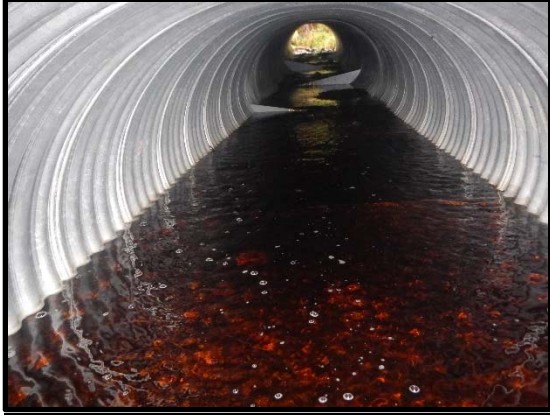
Culvert barrel, looking upstream 2017
