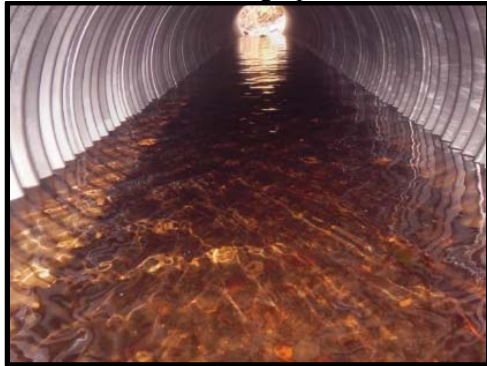
Culvert barrel, looking upstream
