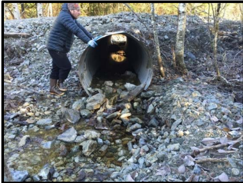
Culvert outlet, looking upstream, 2015
