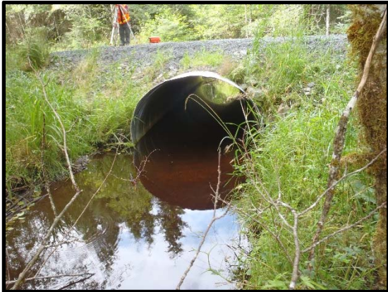
Culvert outlet, looking upstream 2016
