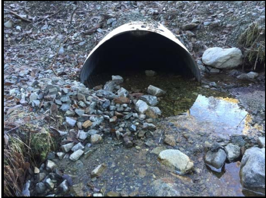
Culvert outlet, looking upstream 2015
