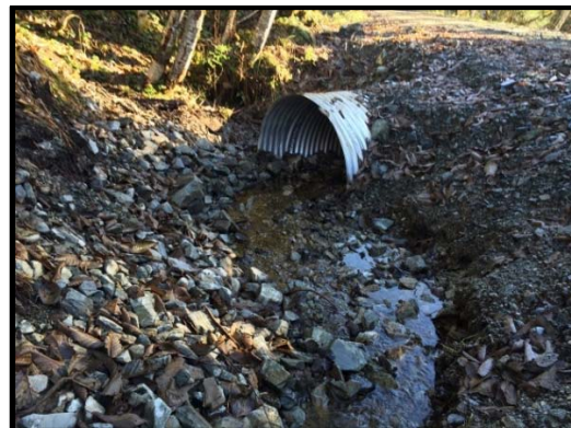
Culvert inlet, looking downstream 2015
