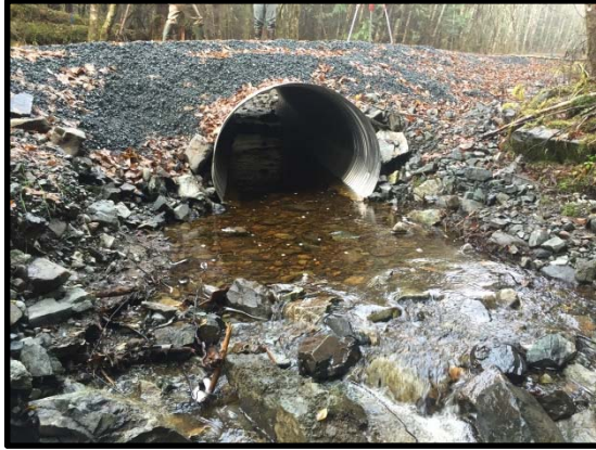
Culvert outlet, looking upstream 2015
