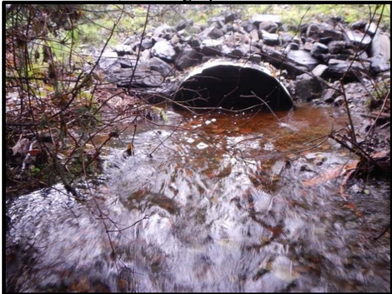
Culvert outlet, looking upstream
