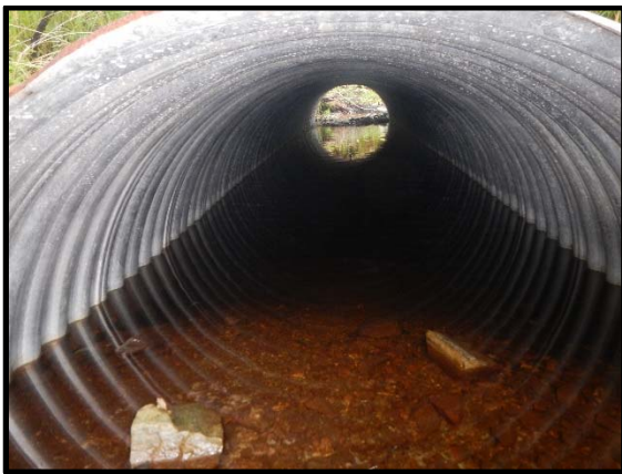
Culvert barrel, looking upstream 2017
