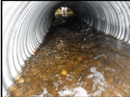
Culvert barrel looking downstream 2015
