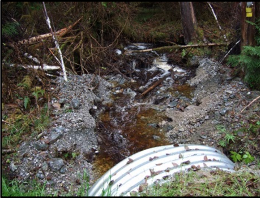
Photo 3. SSS designed culvert with surcharge material upstream of culvert
