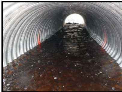
Culvert barrel, looking upstream 2015
