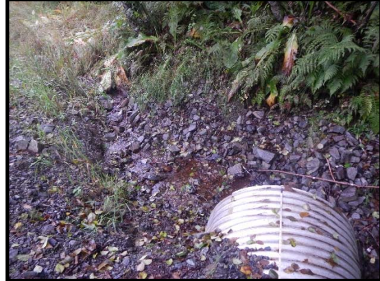
Culvert inlet, looking upstream 2017
