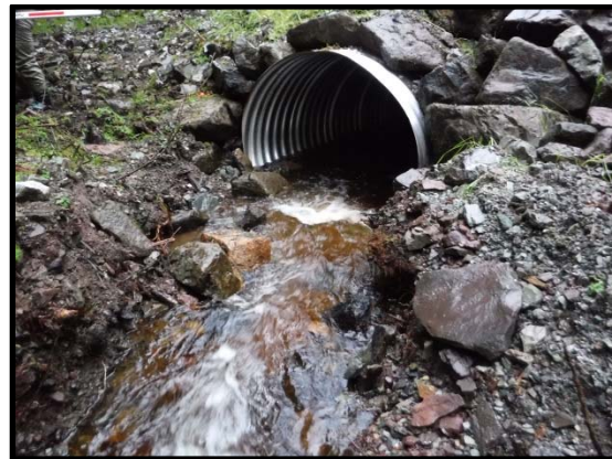
Culvert inlet, looking downstream 2015
