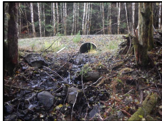
Culvert outlet, looking upstream 2017
