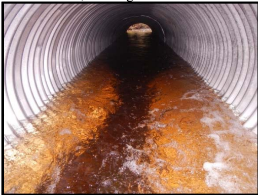
Culvert barrel, looking downstream
