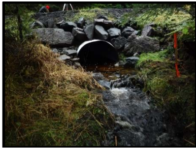
Culvert outlet, looking upstream 2015
