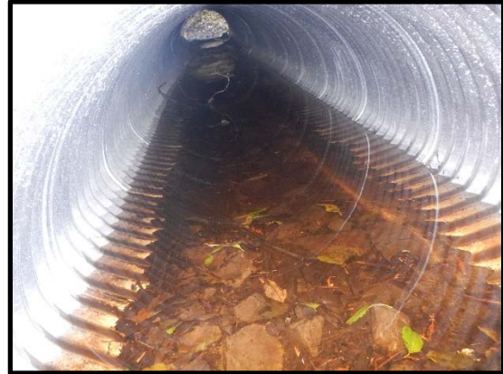
Culvert barrel, looking upstream 2017
