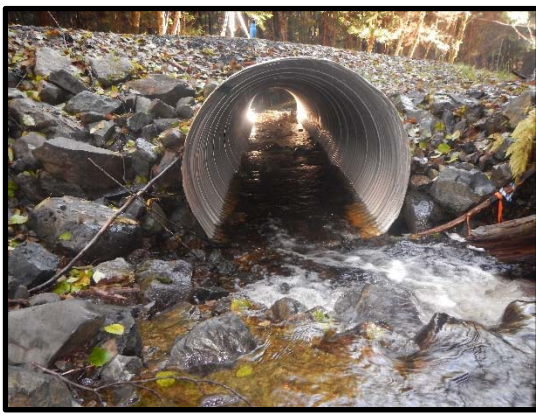
Culvert inlet, looking downstream 2017
