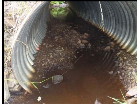
Culvert barrel looking downstream 2016
