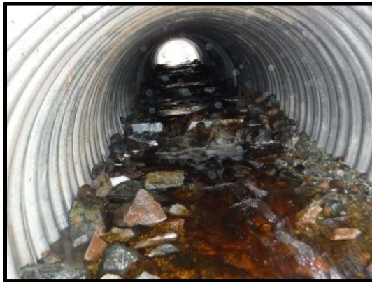
Culvert barrel, looking upstream 2015
