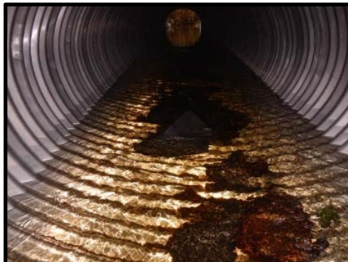
Culvert barrel, looking downstream
