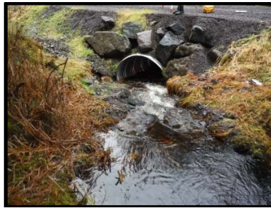
Culvert inlet, looking downstream 2015
