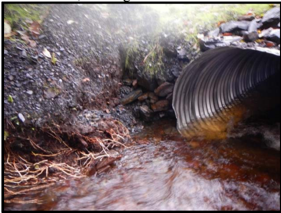
Culvert inlet, looking downstream
