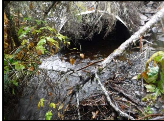
Culvert outlet looking downstream, 2015
