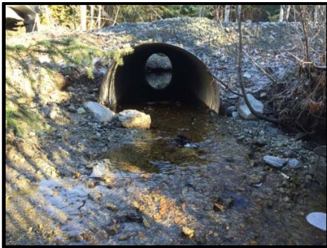
Culvert outlet, looking upstream 2015
