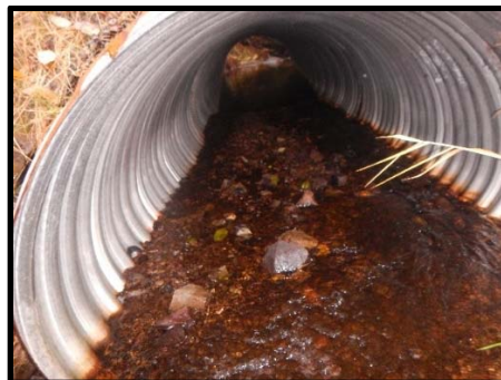
Culvert barrel looking downstream 2017
