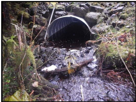
Culvert outlet, looking upstream 2017
