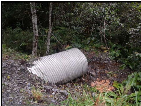
Culvert outlet, downstream 2017
