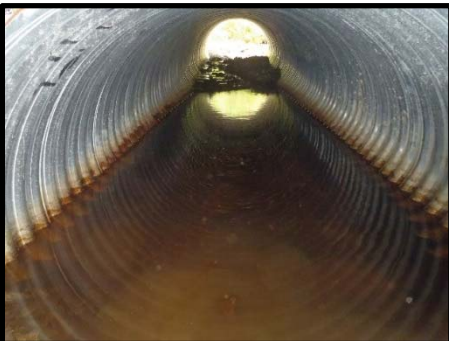
Culvert barrel looking upstream
