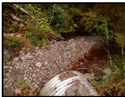
Culvert inlet, looking upstream 2017
