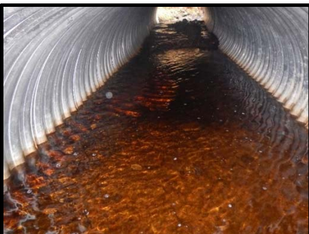
Culvert barrel looking upstream
