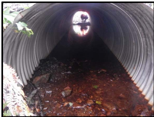
Culvert barrel, looking upstream 2017
