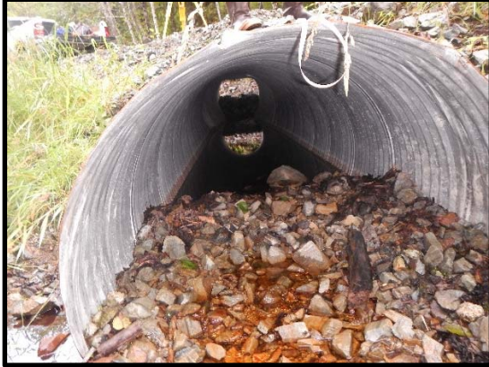
Culvert barrel, looking upstream 2017
