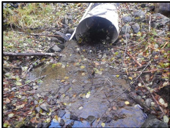
Culvert inlet, looking downstream 2017
