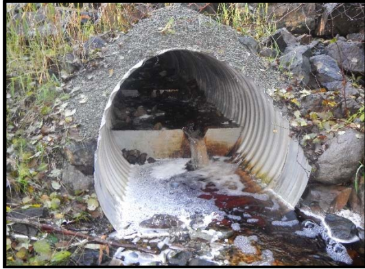
Culvert outlet, looking upstream 2017
