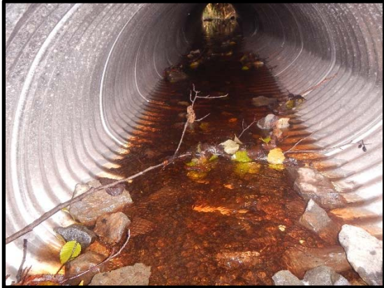
Culvert barrel, looking downstream 2017
