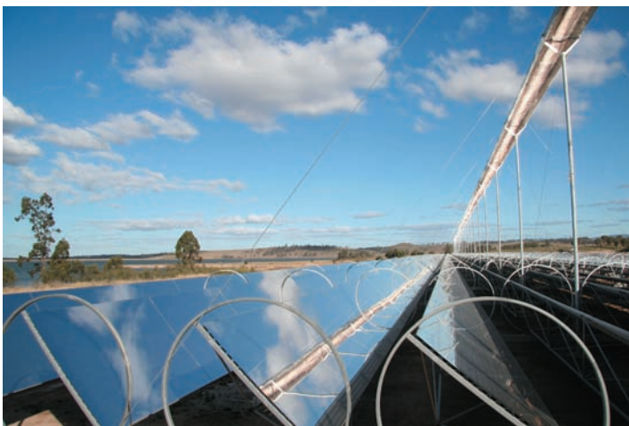
Compact Linear Fresnel reflectors and linear receiver. (Photo courtesy of Areva Media Department)
