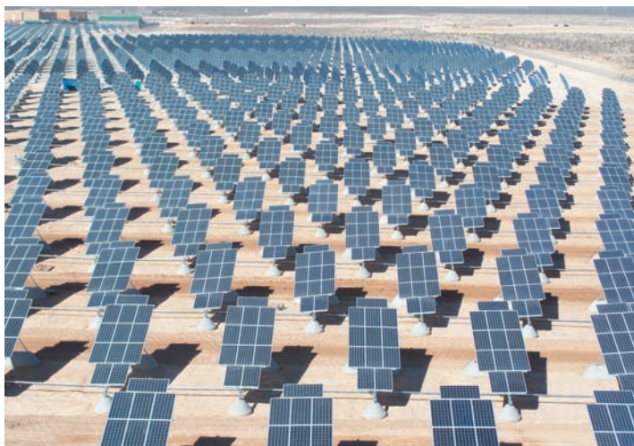
Nellis Air Force Base in Nevada is home to a PV system with 72,000 solar panels that produce 14 MW of electricity. (U.S. Air Force photo by Airman 1st Class N. Y. Barclay)
