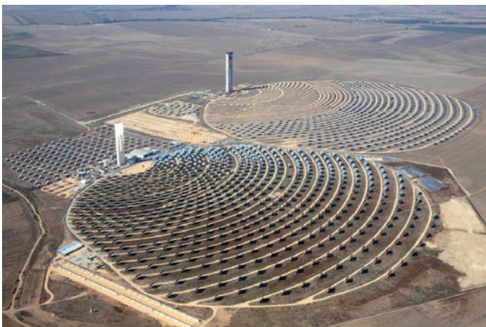
Abengoa's PS10 and PS20 power towers near Seville, Spain use reflectors that track the sun to concentrate the sun's energy to a focal point in the tower where liquid is heated to > 1,000° F and used to generate electricity.
