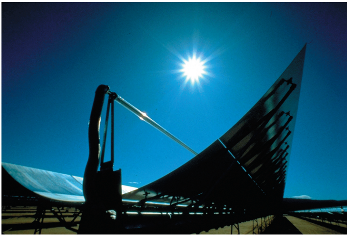
A Parabolic Trough System uses a reflective trough to heat a tube filled with oil to produce steam to drive a turbine to generate electricity. (Photo courtesy of Sandia National Laboratory)
