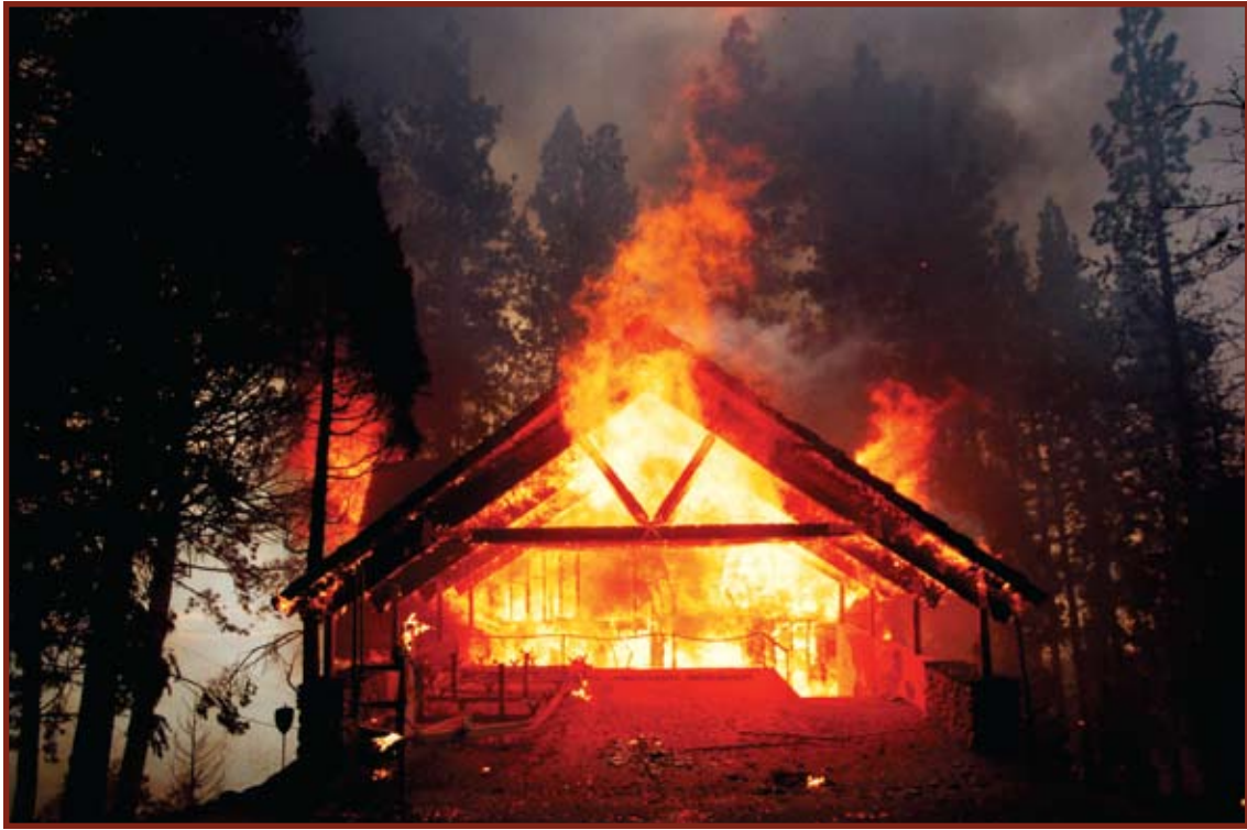
Figure 6. Typically in the subdivisions, the homes were burning and the adjacent vegetation was not. (Photo by Brett Snow, San Bernardino Sun)
