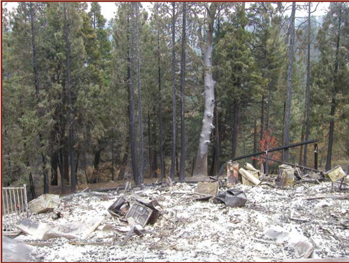
Figure 16. Note the unburned vegetation adjacent to the burned structure. The scarring on the tree indicates the tree caught fire from the structure and not the reverse.
