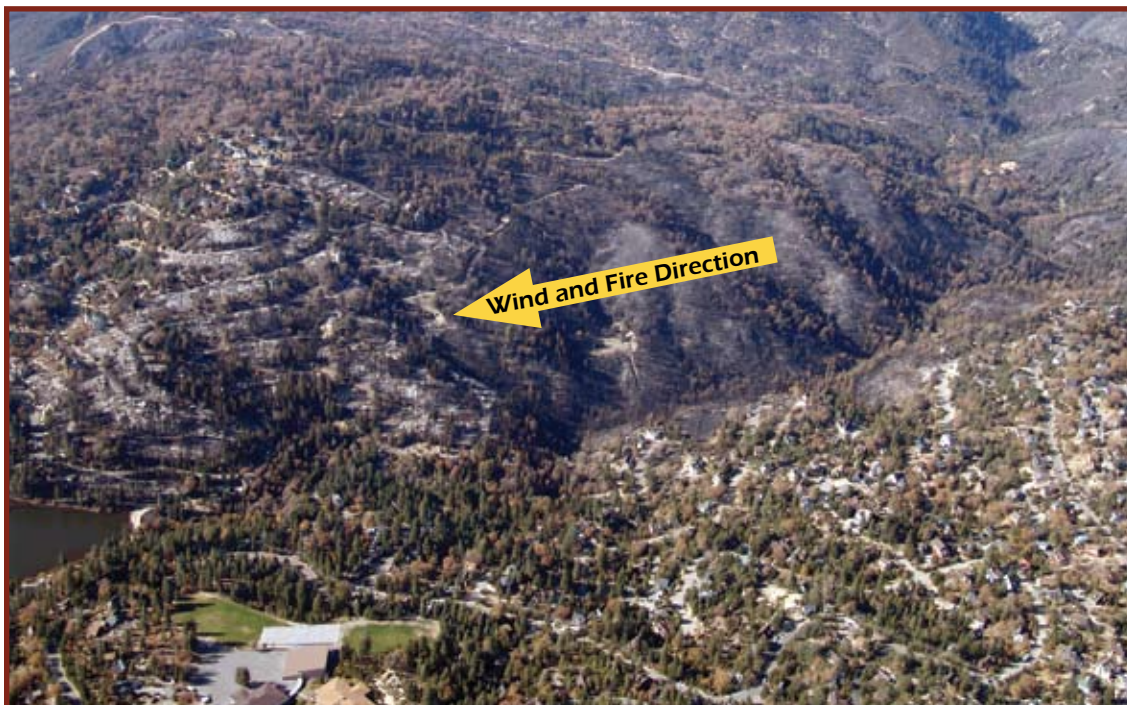
Figure 12. Consecutive burned homes where streets were aligned with the wind are indicated by the arrow.
