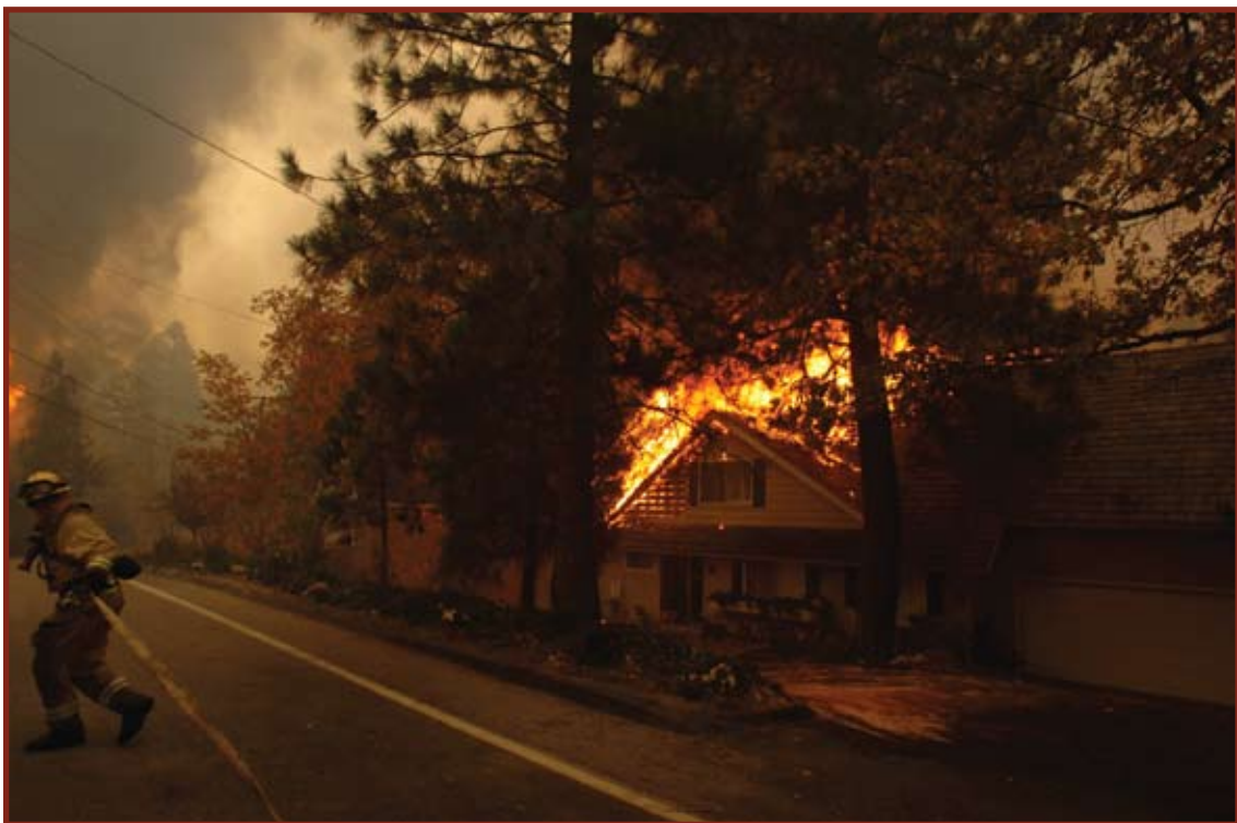
Figure 7. Flammable roofs were vulnerable to embers. (Photo by Eric Reed, San Bernardino Sun)
