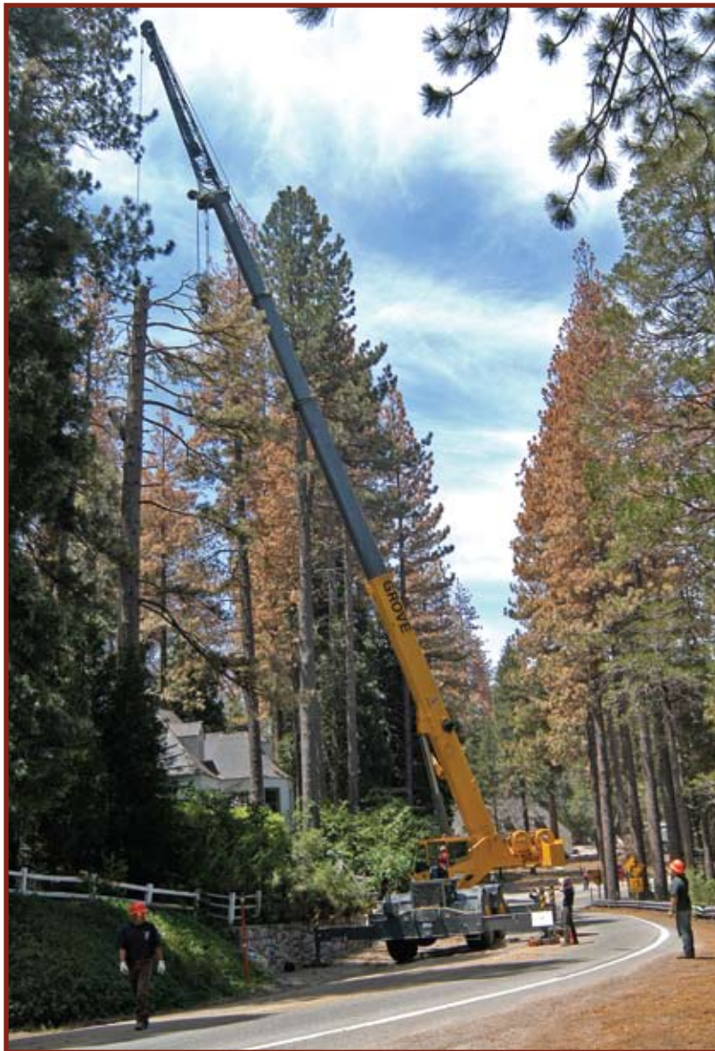
Figure 20. Large dead tree removal on private property.
