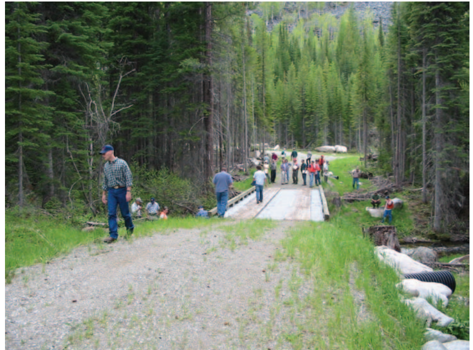
Figure 1. BMP teams inspect road drainage and erosion control on a bridge approach during a calibration exercise before the 2004 audit. (Photo provided by Brian Sugden.)
