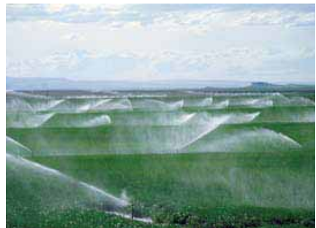
Handline sprinkler irrigation system – United States 2000
