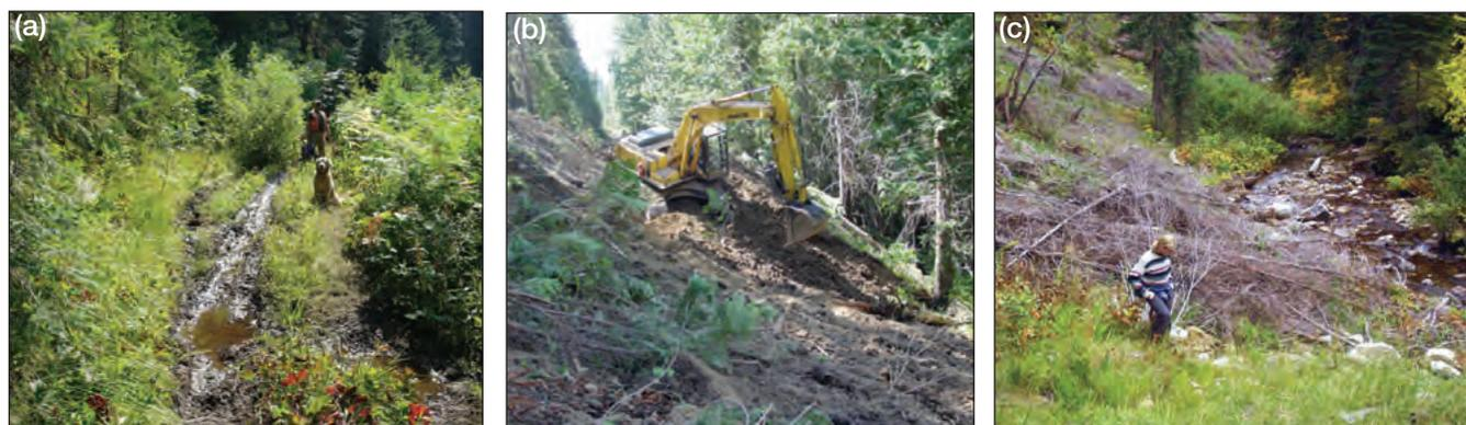
**Figure 2.** Abandoned roads (a) before recontour, (b) during recontour, and (c) 3 years after recontour.
