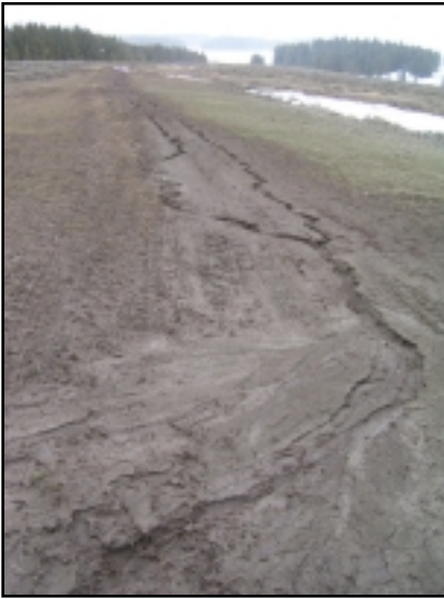
The Oil Well road is used by ORV's traveling into the Cabin Creek WMA. Snowmobiles and 4-wheelers have denuded the meadows along the trail and led to this erosion, documented in April 2003/ Photo by Phil Knight.
