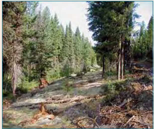
Figure 39—In this project on the Lolo National Forest in Montana, the original road paralleled a stream channel that often eroded portions of the road, delivering large volumes of sediment to the stream. Through a stewardship timber sale contract, a new road was built away from the stream, and the old road was decommissioned.
