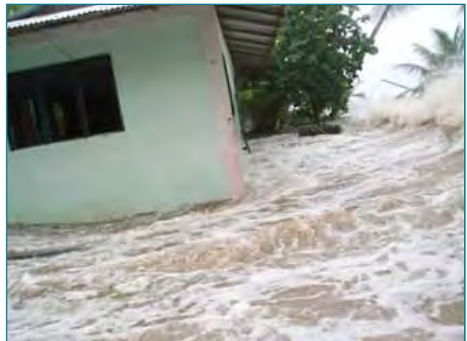
Figure 27—In the winter of 2007 and again in 2008, coastal communities throughout the Federated States of Micronesia (FSM) experienced abnormally high tides that flooded homes, washed out beaches, and undercut and damaged roads and other infrastructure. Such events are expected to become more frequent and destructive, as sea level rises and storms intensify.
