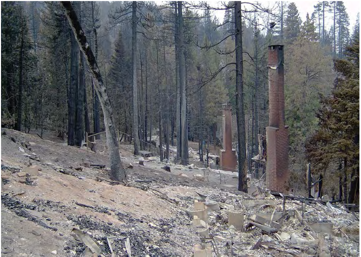
This is a typical WUI fire disaster scene with unconsumed and green vegetation surrounding burned structures (Grass Valley Fire). The homes ignited from low-intensity surface fires and firebrands (lofted burning embers). The trees then caught fire from the burning homes. The totality of destruction is due to the lack of fire suppression rather than the intensity of the initial ignition sources.
