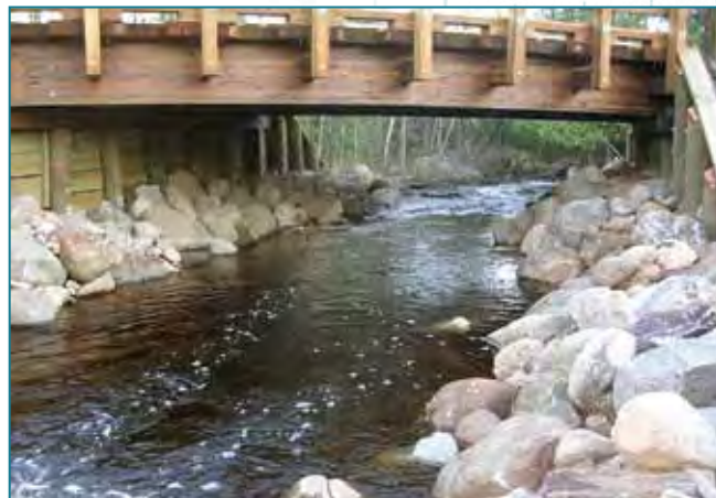
Figure 34—Restoring fragmented flow paths and habitats on the Chequamegon-Nicolet National Forest. At Armstrong Creek Crossing, five undersized culverts in various stages of disrepair (photo on left) were replaced with a 30-foot (9-meter) clear span wooden bridge (photo on right). The culverts, which had a total waterway opening of 24.5 square feet (2.3 square meters), would fill to capacity during a 2-year flood; the road would overtop during a 100-year flood. The realigned crossing restores flow to a meander that was abandoned when the culverts were installed, restores fish passage for brook trout, and improves habitat connectivity for other aquatic organisms. With a waterway opening of 200 square feet (19 square meters), the new structure can accommodate flood flows in excess of the 500-year flood and enable the stream to function more naturally during large runoff events. For additional examples, see http://www.stream.fs.fed.us/fishxing/case.html .
