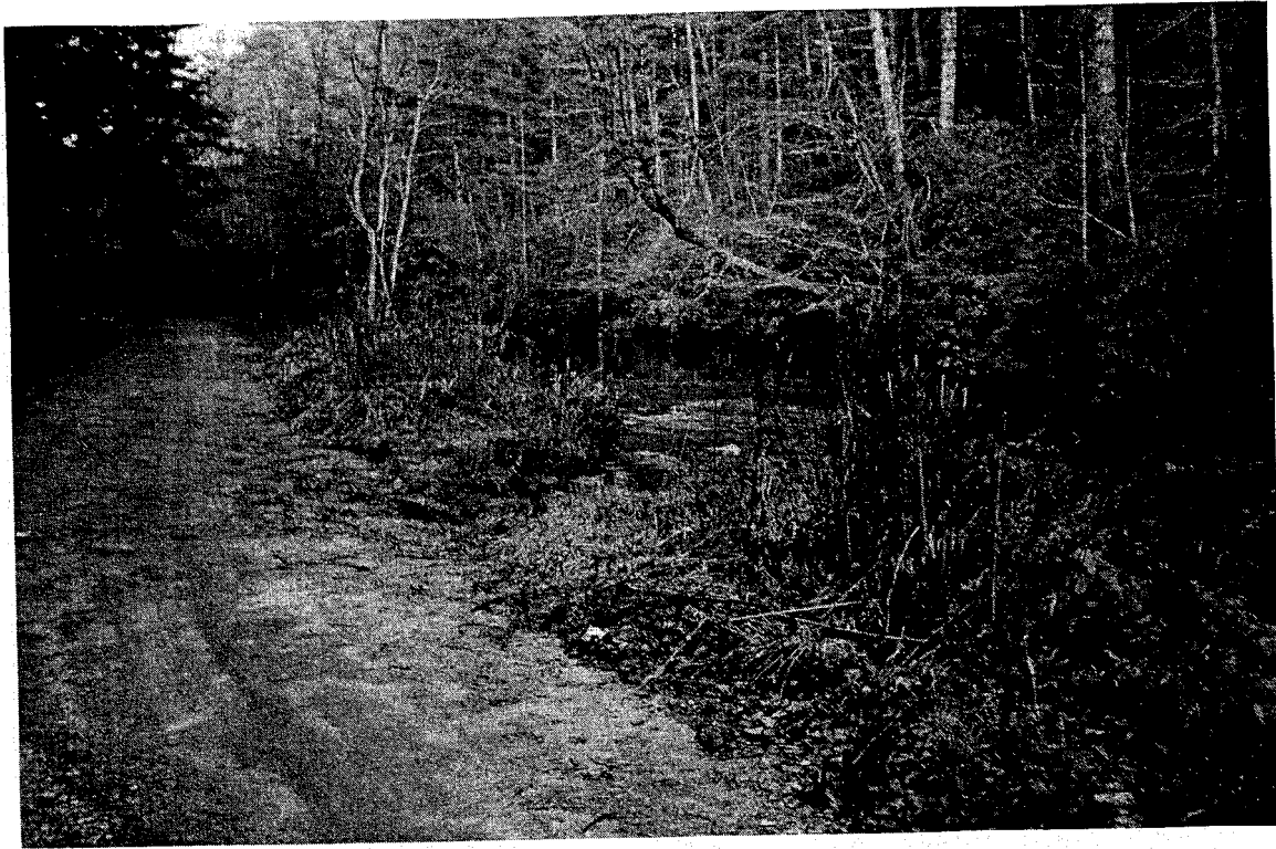
Figure 6. Location of unpaved road adjacent to Warwoman Creek—break in road berm allows sediment to enter directly into creek.
