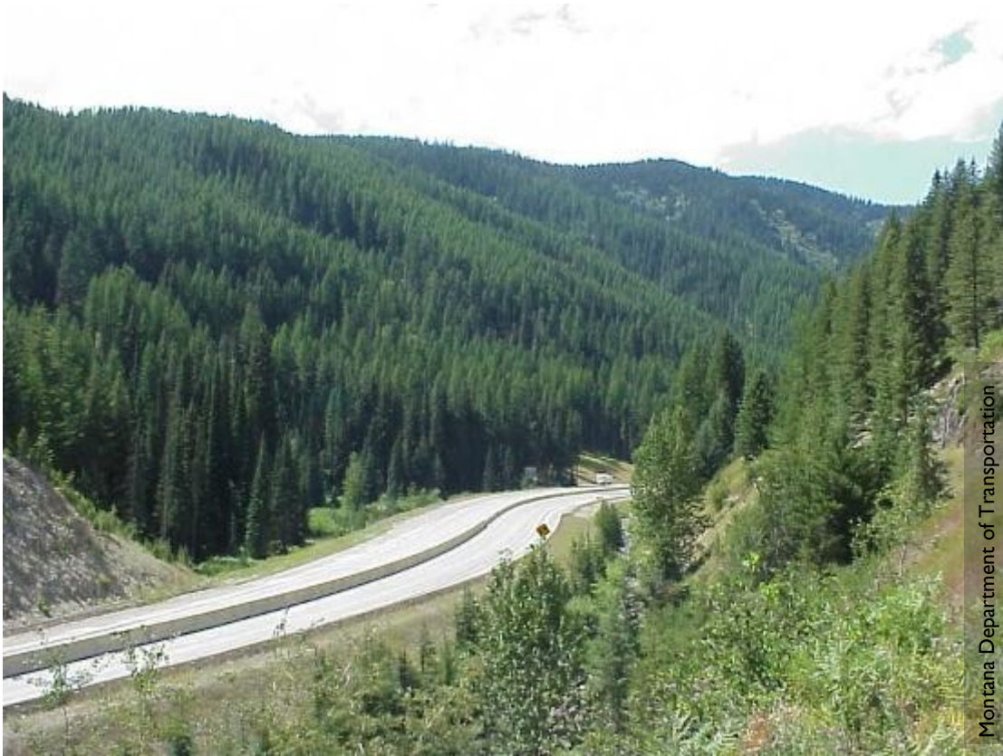
Plate 4.5. Jersey barriers in the medians or along the shoulders of highways and fenced areas adjacent to highways may impede movement of lynx between habitat patches.
