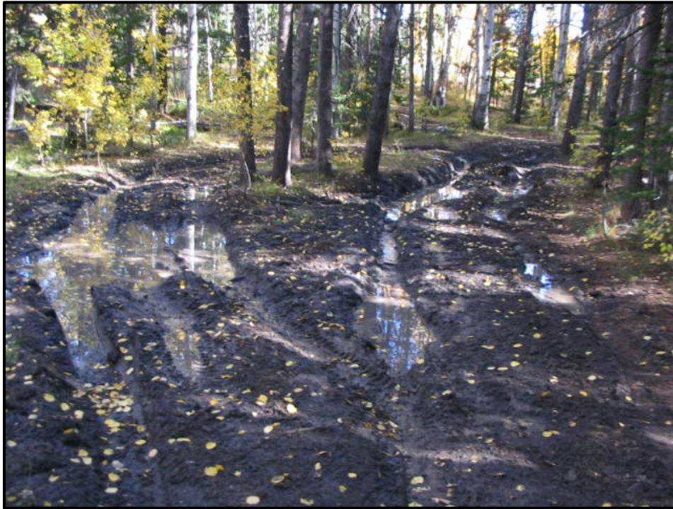
Figure 24. National Forest System Road 803.3F is proposed for decommissioning due to its location along an ephemeral stream and the deep ruts that contribute to degradation of water resources. Addition of an unauthorized route in a better location to the southeast would provide improved access to this area of the forest.
