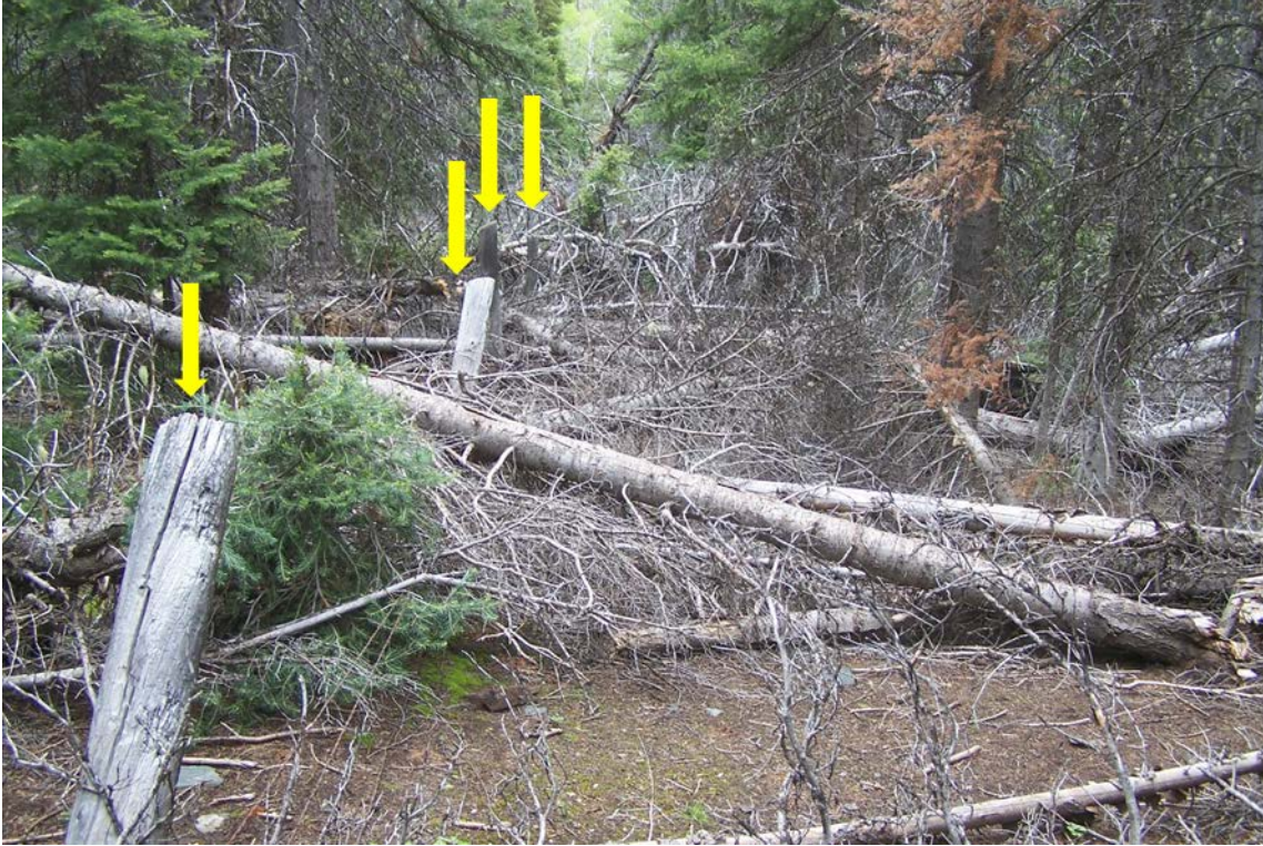
Figure 19. Deadfall across post and wire boundary fence in the Jack Creek Allotment. Yellow arrows indicate fence posts.
