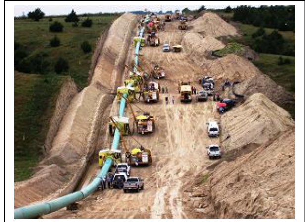
Figure 1.5-1 – Leveled work corridor for pipeline installation, showing cut hillsides and dewatering. Heavy equipment and truck traffic, along with soil stockpiles, will compact soils.
