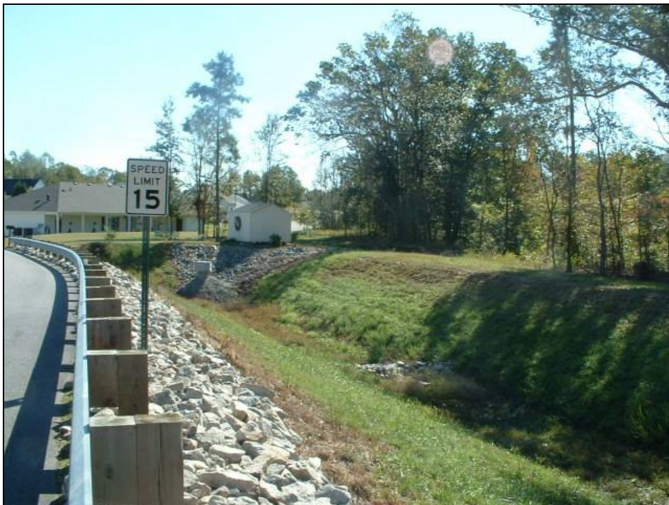
Dry detention basin. Source: http://www.colonial-heights.com/assets/images/009.jpg
