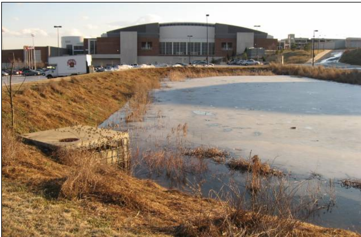
Wet pond receiving stormwater runoff from parking lots serving the Comcast Center sports arena and other facilities at the University of Maryland, College Park. Emergent wetland
