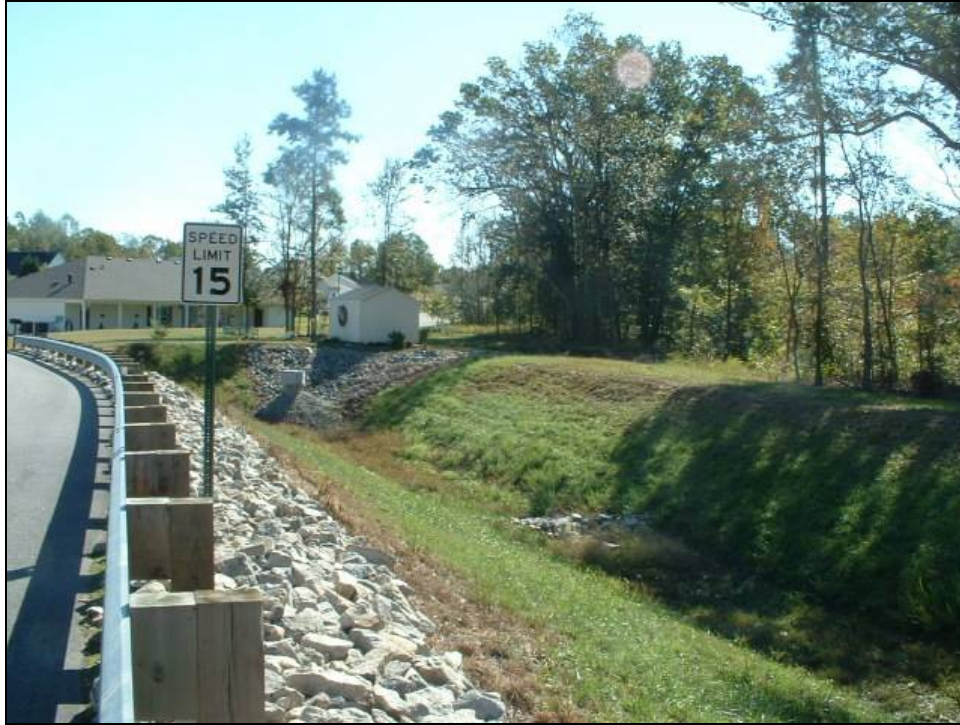
Dry detention basin. Source: http://www.colonial-heights.com/assets/images/009.jpg
