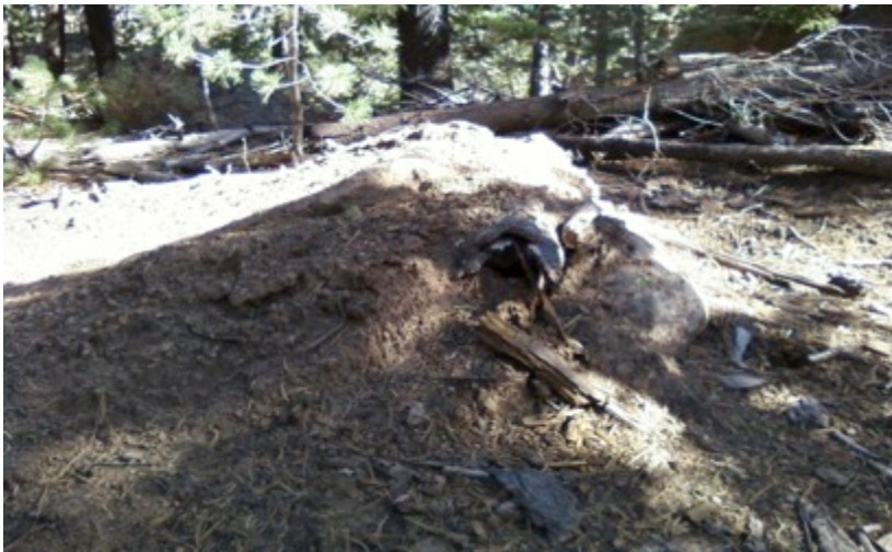
Figure 6 Illegal trail construction. Photo by Emma Benenati.
