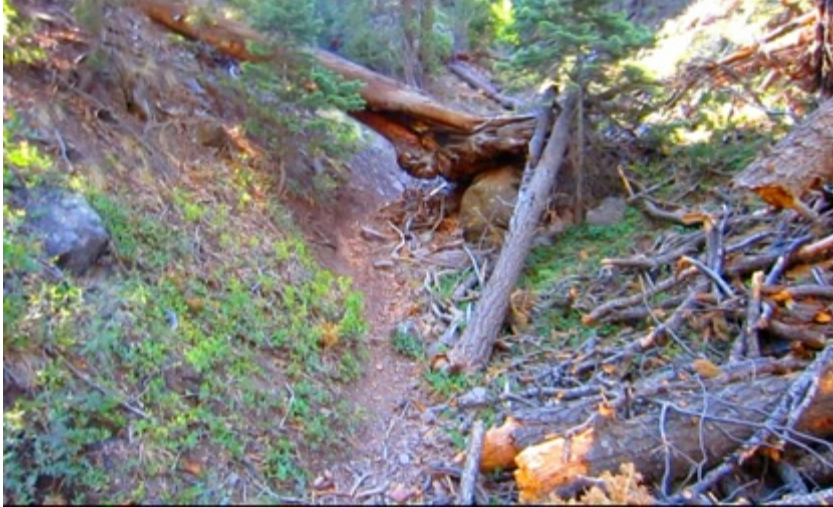
Figure 5 Illegal trail construction. Photo by Emma Benenati.
